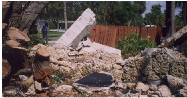
Hurricane Wilma destruction, ROH entrance on Camino Real, 2005
